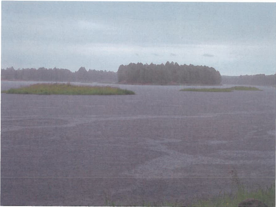
Artificial islands below the bridge.
